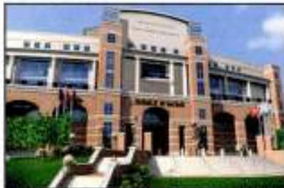
This image shows what the front of the finished stadium will look like. (WFU Illustration)
